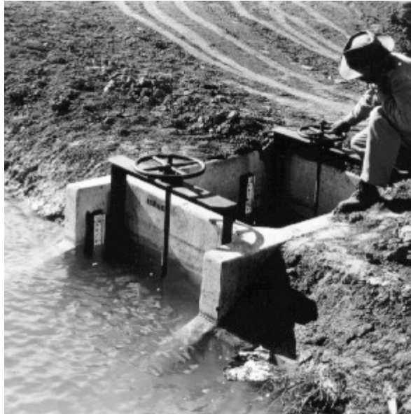
Figure 9-3 -- A single-barrel CHO turnout.
