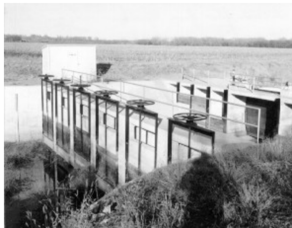
Figure 9-7 -- Gated orifice check structure used to maintain upstream water surface levels and to measure rates of flow in the Courtland Canal, Nebraska.
