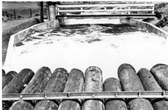
Figure 5-4 -- Turbulence and waves in a Parshall flume produced by an outlet works stilling basin. The log raft failed to quiet the flow.
