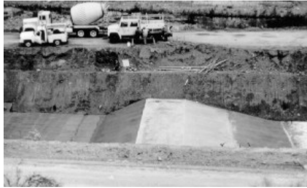
(a) Long-throated flume (broad-crested weir) under construction.
