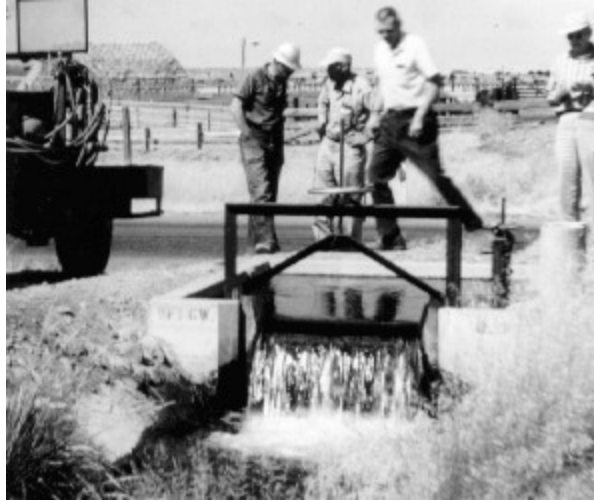
Figure 7-14 -- Adjustable Cipolletti weir in a division box.
