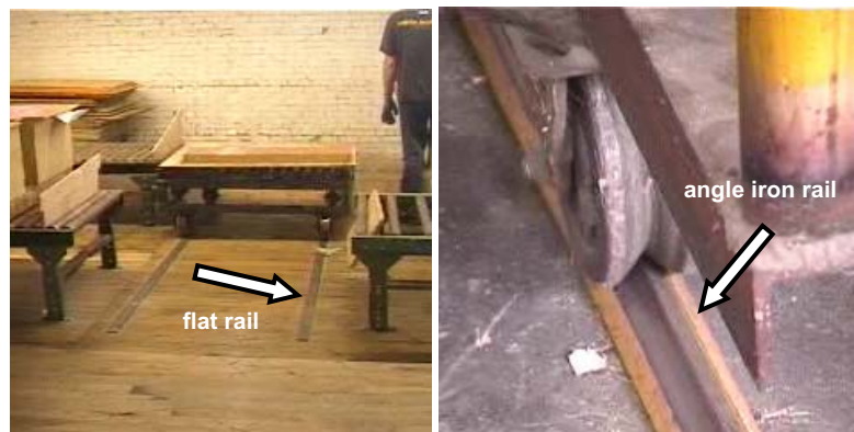
Photo 10. Cart on flat rail design (left); cart wheel on improved angle iron rail system (right).
