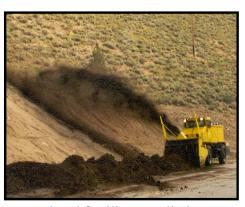
calculations assumed: use of a four-man mulching- machine, seed and fertilizer applied at a rate of 0.75 tons/acre (0.15 metric tons/ha), and an application rate of 2 tons/hour.
