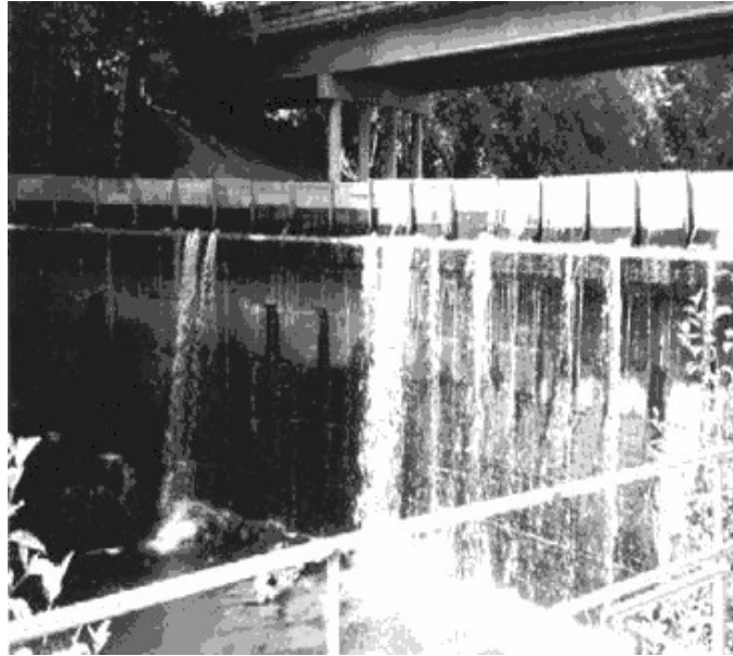
Figure 4-13. Photograph of Hemlock Dam with low flashboard configuration, Skamania County, Washington.
