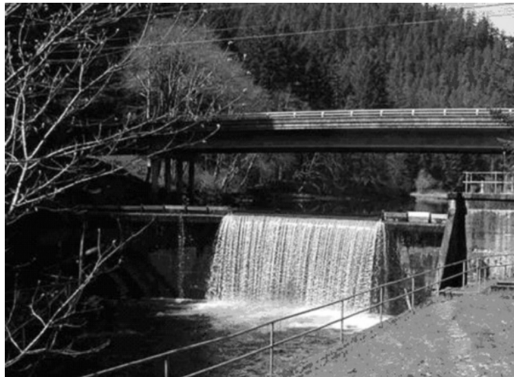
Figure 4-12. 2001 Photograph of Hemlock Dam with the high flow flashboards in place, Skamania County, Washington.
