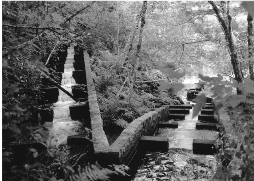
Figure 3-36. View of fish ladder, looking west. USFS photograph, taken 1992.
