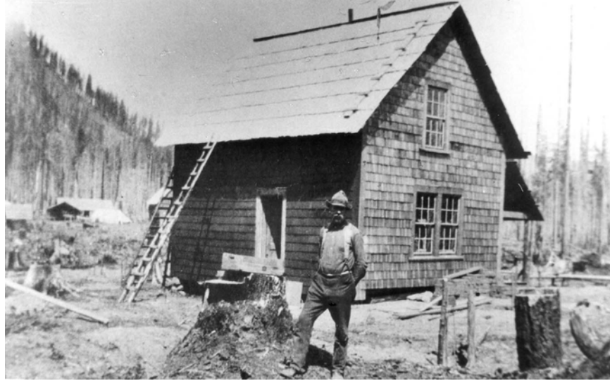
Figure 3-34. Hemlock Ranger Station, constructed on the south side of Trout Creek in 1909 by Ranger E. J. Wigal. Camp 3 visible in background.
