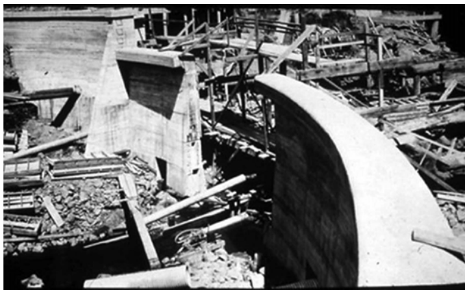
Figure 3-20. 1935 photograph of Hemlock Dam under construction, Skamania County, Washington.
