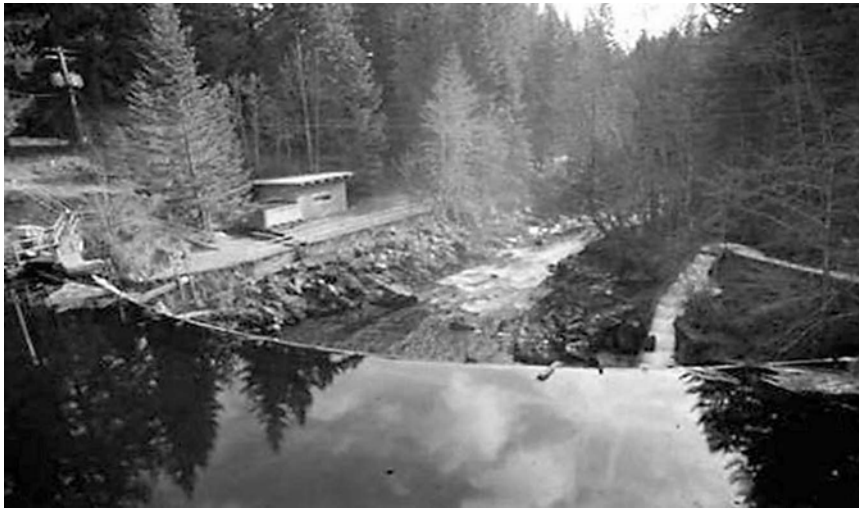
Figure 3-21. 2001 photograph of Hemlock Dam looking downstream from the reservoir, note the fish ladder on the right side of the photograph. Skamania County, Washington.
