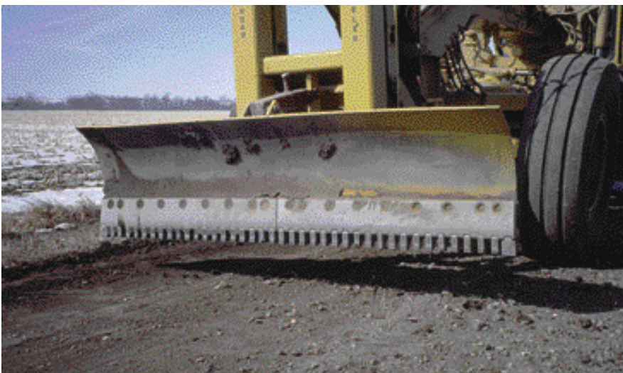
An effective tool for dealing with washboard areas is the front dozer equipped with carbide bits.
