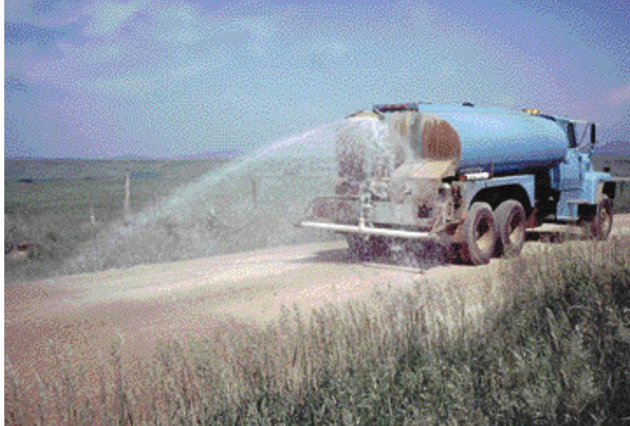
A water truck being used to prewet some very dry gravel just prior to treatment. This dramatically improves the success of the treatment.
