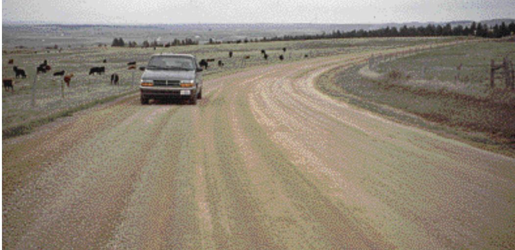
This superelevated road section makes driving safer.
