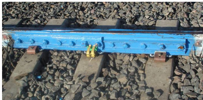
Figure 1. Miter Cut Insulated Joint.
