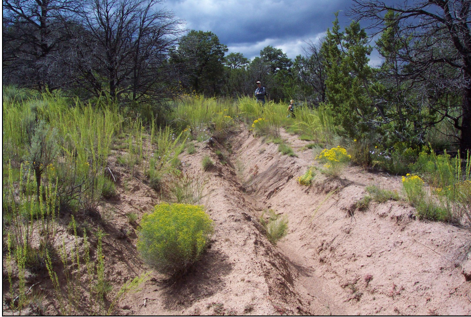
Figure 9. Heavily eroded trail segment 4-E.
