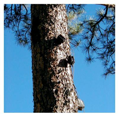
Fig. 5-26. Double Strain Insulators. This medium-sized ponderosa with two strain insulators is located near the bottom of Pueblo Canyon. The line jumped to the south rim of Pueblo Canyon where there was a second tree with a strain insulator to help support the line under stress. (GPS waypoint PC12)
