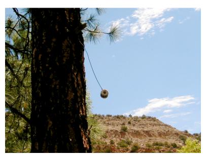
Fig. 4-5. Split Forestry Knob. Porcelain insulator hangs at end of wire in Frijoles Canyon near Headquarters. The telephone wire would have passed through the center hole of the insulator. (GPS waypoint HQ4)
