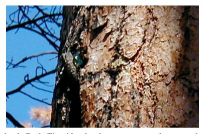
Fig. 5-3. Bracket in Bark. The oldest insulators were sometimes completely enveloped by the bark of the tree. Just the threaded tip of the foot-long wood bracket and a piece of blue glass are all that's visible on a ponderosa in Rendija Canyon. (GPS waypoint R15)
