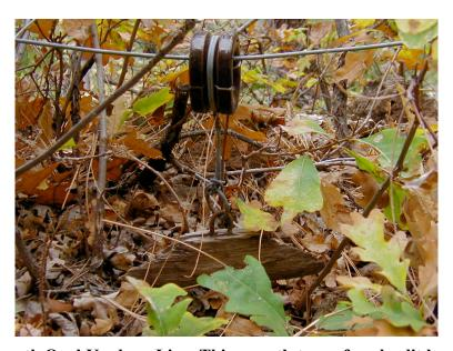
Fig. 5-28. Smooth Oval Knob on Line. This smooth type of oval split knob was found along the Duran Road where it climbs out of the south side of Los Alamos Canyon. The thimble and staple have pulled out of the tree, taking a wedge of wood with them. A long length of telephone line, edging the old road, is still strung through the split knob's center hole. (GPS waypoint D36)
