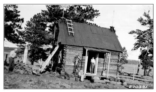
Fig. 2-6. Cerro Valdez Lookout in the Jemez Forest. Located near the town of Coyote, the log cabin roof has two lightning arrestors and the telephone is "posted" outside in a pile of stones. (Photo: U.S. Forest Service)
