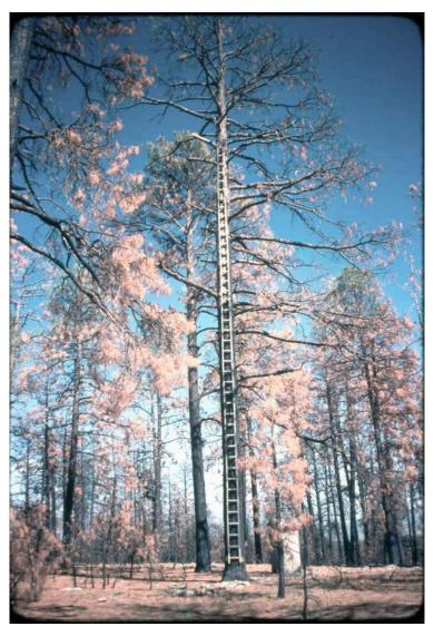
Fig. 2-12. Lookout Tree Ladder at the Wye Upper Crossing. In 1936–7 the Civilian Conservation Corps (CCC) built two ladder trees to help locate fires. One ladder tree was at Upper Crossing (above) and a similar ladder tree was at Corral Hill. Neither ladder tree remains. The CCC also extended the telephone lines to each of the Lookout trees. This photo was taken soon after the 1977 La Mesa Fire. (Photo: Chris Judson, National Park Service)
