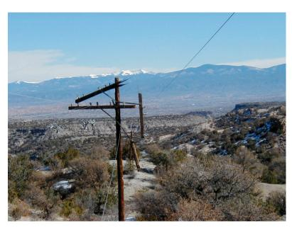
Fig. 5-42. Broken Arms of the Mountain States. It once carried twelve wires on two cross arms to bring phone and telegraph service to Los Alamos.
