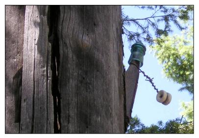
Fig. 4-7. Hemingray with RT&SCO. This appears to be a transition between the Hemingray No. 9 and the small round split knob found on the spur line to Cerro Pelado Lookout—a line originally constructed in 1914. (GPS waypoint AP6)
