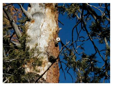
Fig. 5-38. Oval Split Knob in Otowi Section. This forestry split knob is located in Pueblo Canyon. It may have been part of the Forest Service line built in 1943 to connect Pajarito Cabin directly to Española. (GPS waypoint PU5)
