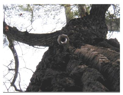
Fig. 4-16. Octagonal Split Knob. This is one of the nineteen octagonal insulators found in Frijoles Canyon near the Upper Crossing Trail. It is attached to the south side of a large cottonwood at north edge of Frijoles Canyon Trail. (GPS waypoint FC6)
