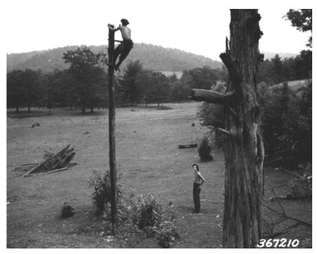
Fig. 3-11. Pole Climbing Practice, 1938. Two CCC boys take turns practicing with climbing spurs used when hanging telephone line. (Photo: U.S. Forest Service)
