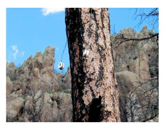
Fig. 5-12. Thomas Flat-sided Oval. Two oval split knobs hang from a large decapitated ponderosa in Cabra Canyon, between the Pajarito Trail and Guaje Mountain. This insulator type was the most common type found on the corridor of the old Pajarito Line. (GPS waypoint PT3)
