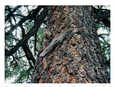
Fig. 5-18. Double Brackets West of Ashley Pond. Two wood brackets are nailed to the north side of a ponderosa in a parking lot west of Ashley Pond and north of Trinity Drive. This tie tree carried two east-west lines. (GPS waypoint BR1)
