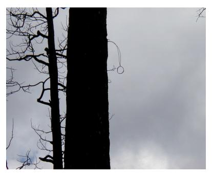
Fig. 5-4. Insulator Loop. An attachment wire with the insulator loop droops from a ponderosa on the old Pajarito Line. While it is evident that this was a porcelain split knob, not a Hemingray, we cannot conclusively identify the type of split knob. (GPS waypoint PT36)
