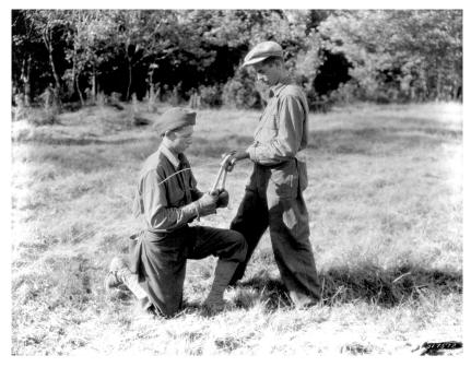
Fig. 3-10. CCC Boys Practice Splicing Telephone Wire, 1935. The new tool crimps lead casing around the two wire ends. The earlier method was the Western Union splice where the two wires were twisted together and the ends tightly wrapped. (Photo: Forest Historical Society, Duke U)
