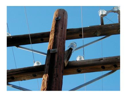
Fig. 5-44. Side Bracket on the Pole Line. The side bracket and insulator may have carried the single Forest Service telephone line that joined the Mountain States pole line in the Otowi section of Bandelier.
