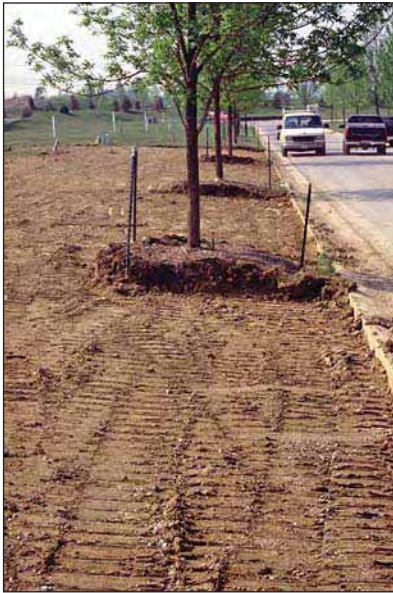
Figure 16. Soil compaction from construction equipment. (Photo by Joe Boggs)
