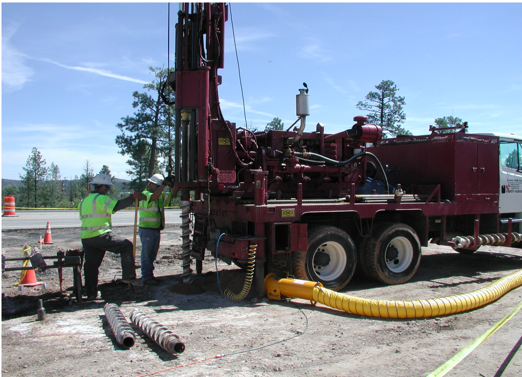
Figure B-18 Installation of borehole location 61-26621
