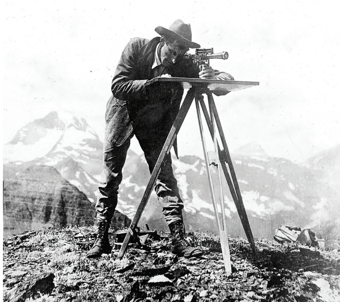
Figure 1. Herbert “Shortie” Clark mapping with a plane table and telescopic alidade in the early 1900s.
