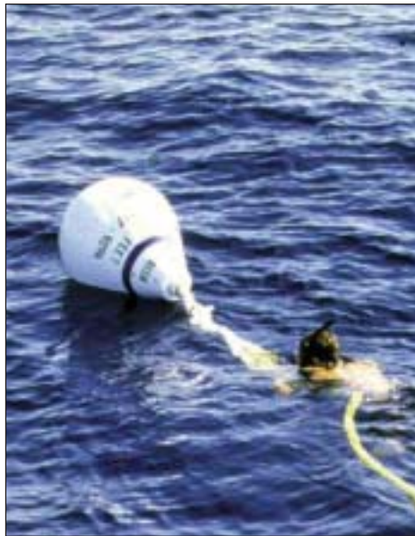
Figure 215. Mooring bouys have been installed at FGBNMS to prevent anchor damage to corals (Photo: Joyce and Frank Burek).
