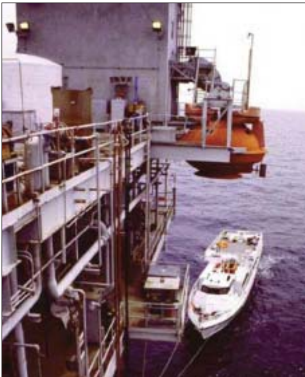
Figure 213. The High Island 389A gas production platform within the Sanctuary (Photo: Frank and Joyce Burek).
