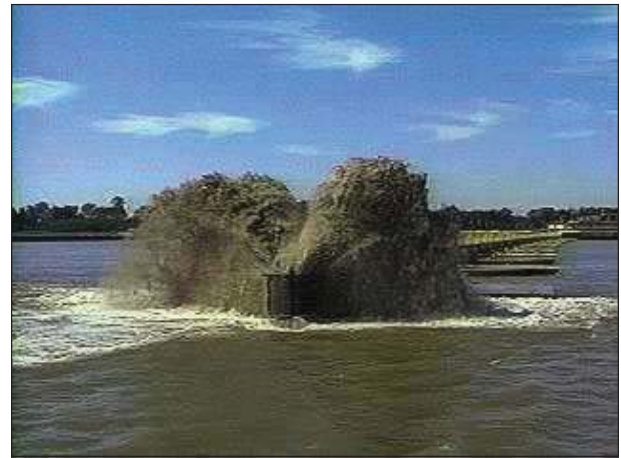
Figure 72. Turbid water from dredging (Photo: National Ocean Service Photo Gallery).
