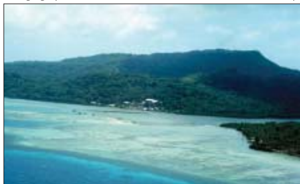
Figure 308. Causeway on Chuuk with remnants of a coral dredging operation from construction (Photo: James McVey).
