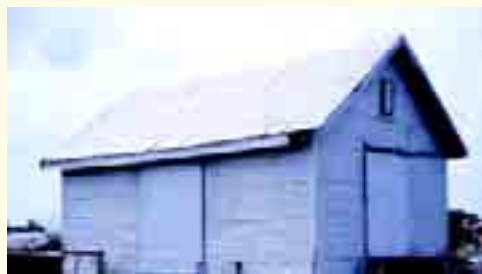
Pesticide storage shed
