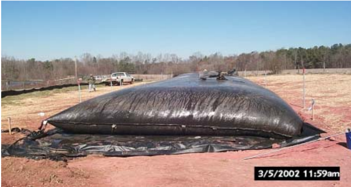
Figure 1. Geotextile Tube on Lined Pad
