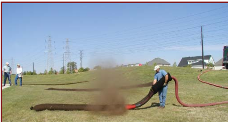
Figure 4. Compost and wood chip mixture applied in a mesh casing as a filter sock to control runoff and sedimentation.
