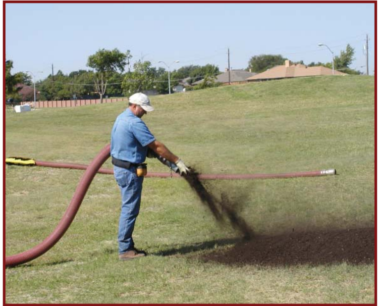
Figure 3: Grass seed and compost being applied as a filter berm in a city park waterway to control runoff and sedimentation.
