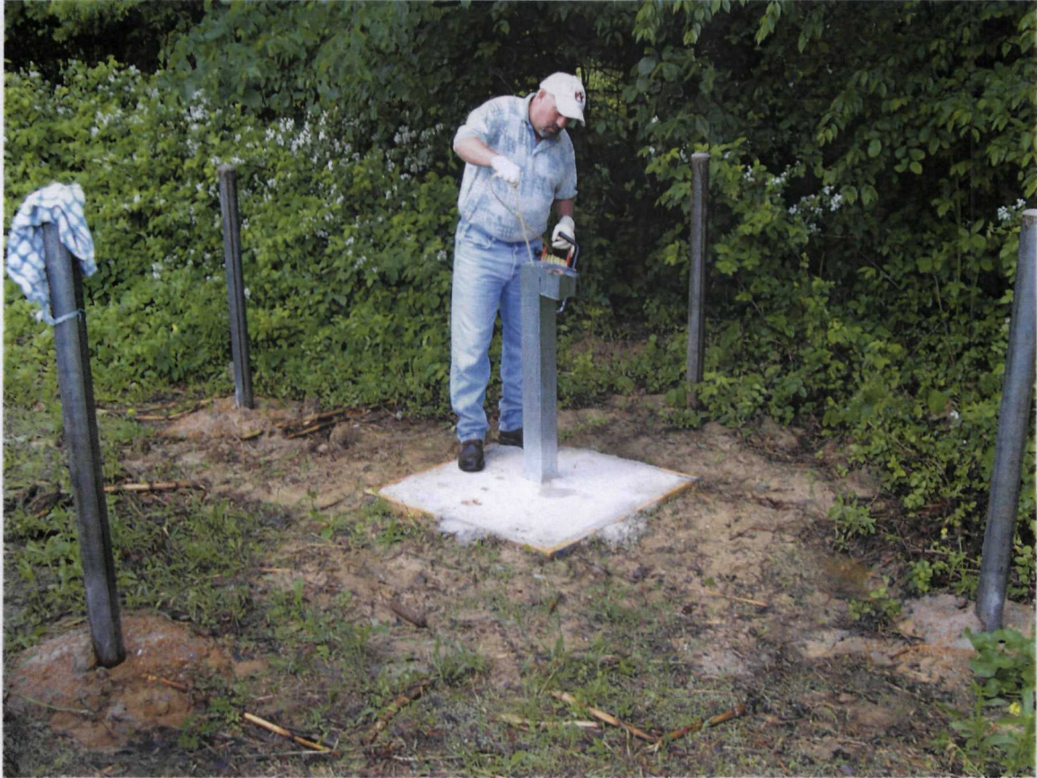
Photograph 6 COP-4 – Jeff Keenum of BAT Associates, Inc. taking a depth measurement at MW-09, newly installed well.
