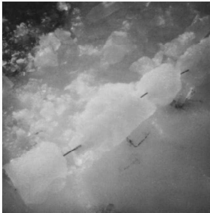
a. ~5 in. on a 0.25-in. guy on the summit of Cadillac Mountain (photo Robert Parker, U.S. Coast Guard).
