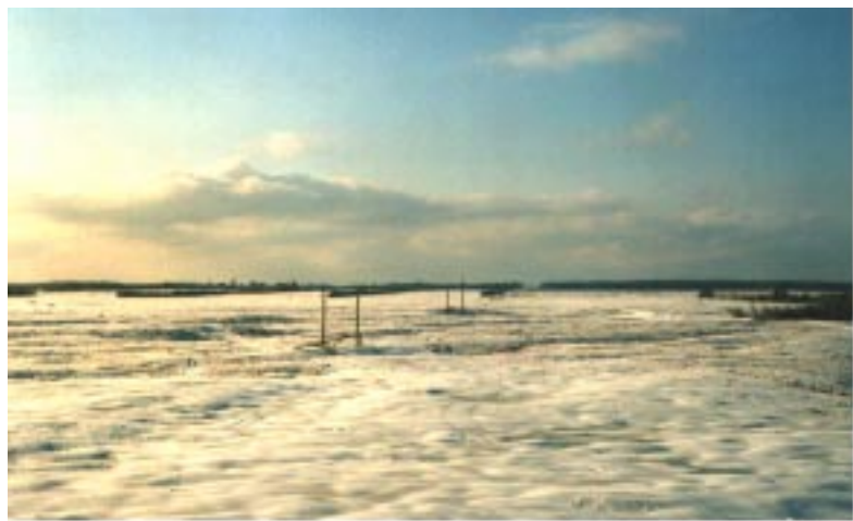
Figure 17. Six miles of Bangor Hydro's 115-kV H-frame transmission line in the blueberry barrens east of Deblois failed under the ice load (photo Larry Billings, Bangor Hydro).
