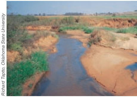
Figure 5. The roots of vegetation act like reinforcing bars to stabilize banks. When vegetation is lost, banks become susceptible to erosion.
