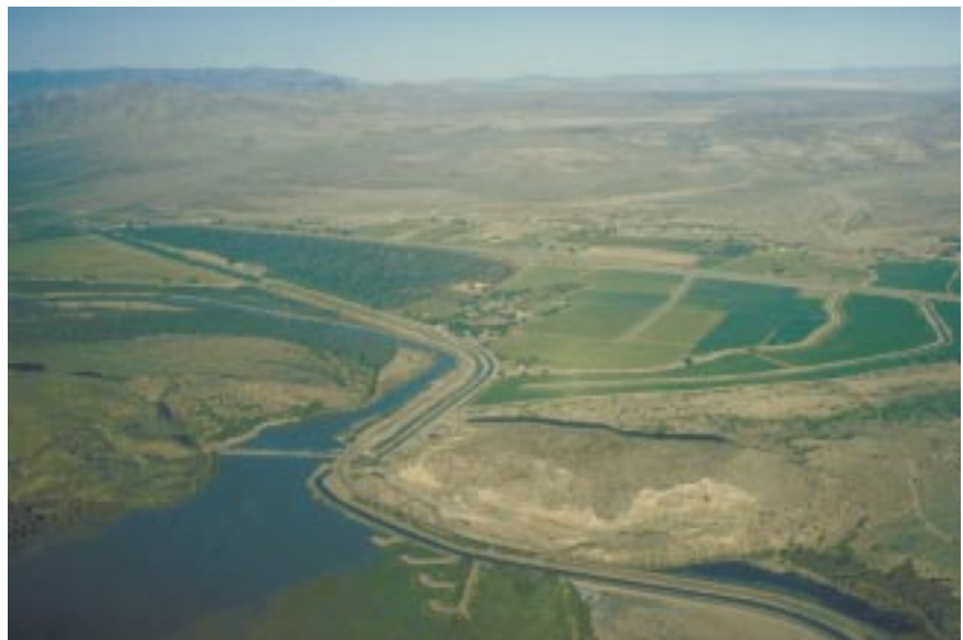
San Acacia Diversion Dam on the Rio Grande about 55 miles downstream from Albuquerque is one of several diversion dams established on the Rio Grande for surface-water irrigation (photograph by Sherman R. Ellis, U.S. Geological Survey).
