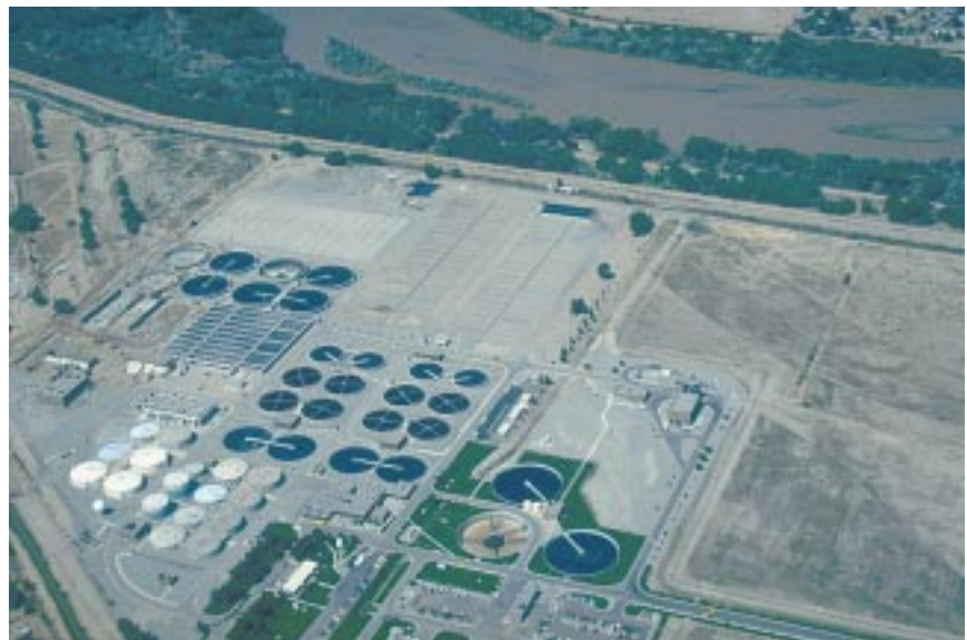
Wastewater-treatment plants affect nutrient concentrations in the Rio Grande (photograph by Sherman R. Ellis, U.S. Geological Survey).
