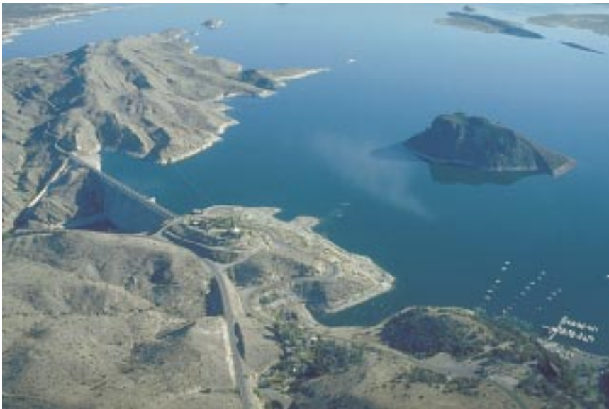
A site in Elephant Butte Reservoir, one of four major reservoirs on the main stem of the Rio Grande, was cored for analysis of selected pesticides (photograph by Sherman R. Ellis, U.S. Geological Survey).
