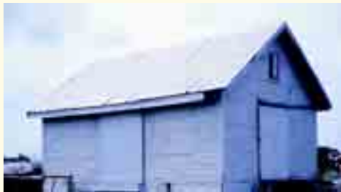
Pesticide storage shed
