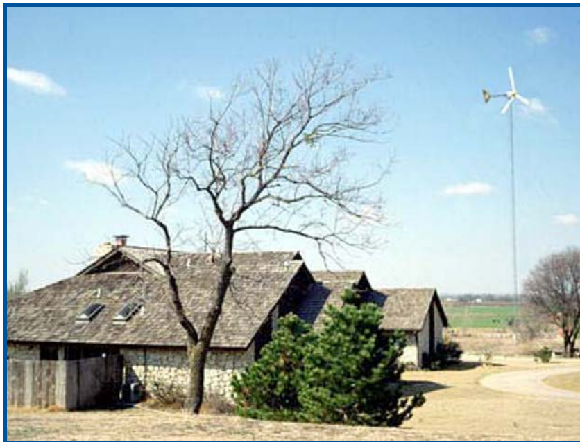
Homeowners, ranchers, and small businesses can use wind-generated electricity to reduce their utility bills. This grid-connected system installed in Norman, Oklahoma, reduces the owner's utility bill by $100 per month. Photo courtesy of NREL.
