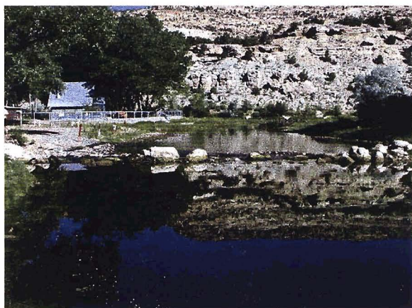
Navajo Dam Water Users Association intake gallery
