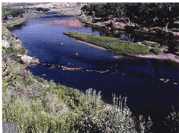
Cottonwood Diversion and intake gallery.
