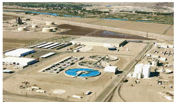
Figure 20 – Aerial Photo of Yuma Desalting Plant.
