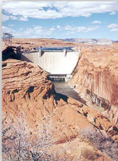
Glen Canyon Dam
