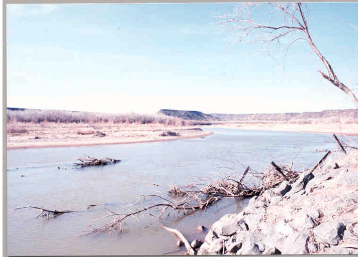
Figure 1. Looking upstream from the project curve. High flows cut into levee eroding the bank. Large gravelbar on opposite bank. Overbank flooding of bar occurs at 13,000 cfs.
