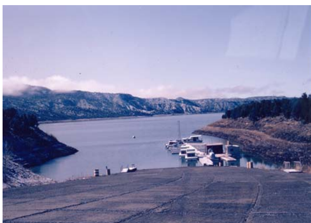
Figure 3-1: Arboles (CO) Boat Ramp, April 1983 (USBR file photo)
