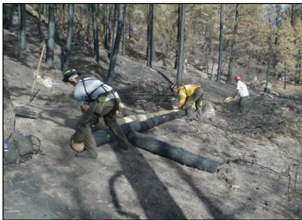
Log Erosion Barrier with Wattle
