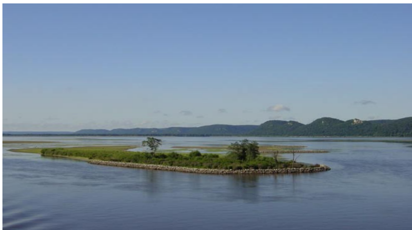
Upper Mississippi River near Genoa, WI. The island picture is a constructed island designed to replace those lost to erosion from lock and dam operations.
