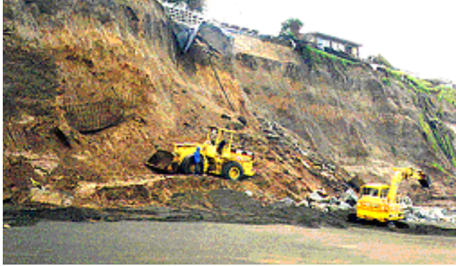
Coastal Cliff Failure along the California Shoreline at Esplanade Beach, Pacifica.
