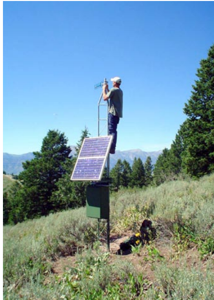
USGS intern David Fee completes the installation of a seismic station in Wyoming, part of the new ANSS Teton Regional Seismic Network in the Jackson-Hole -Teton area.
