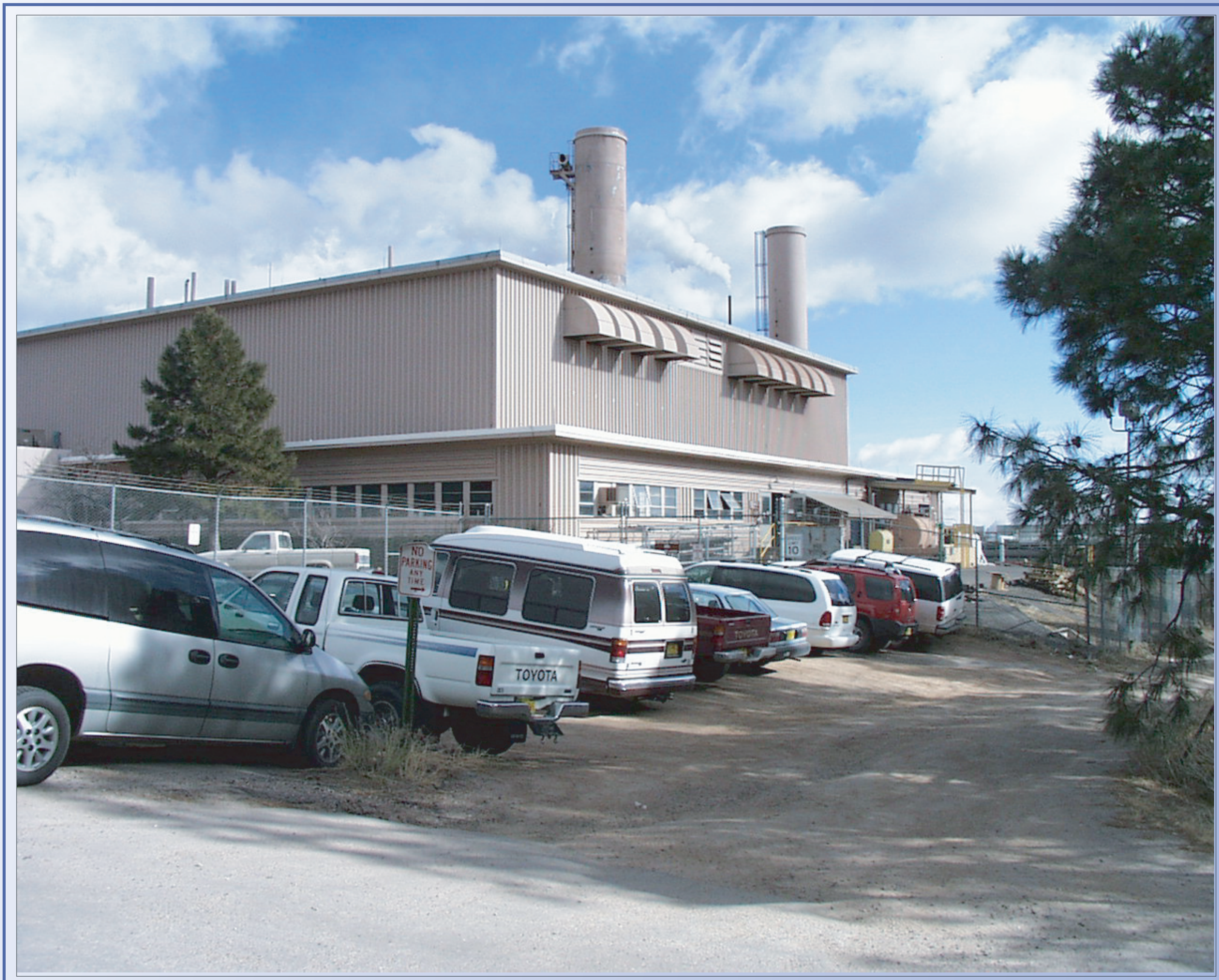
Power Plant at Technical Area 3
