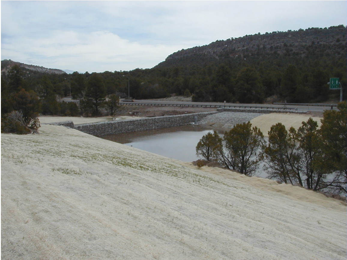
Figure 2.2.2-6. Low-head weir in Los Alamos Canyon retaining snowmelt runoff, April 5, 2001.
