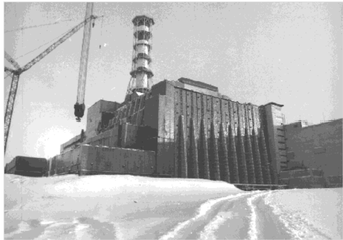
Figure 4-4. A View of the Sarcophagus Covering the Chernobyl Reactor Facility (adapted from http://193.125.172.36/www-kiae/POLYN/history.html )
