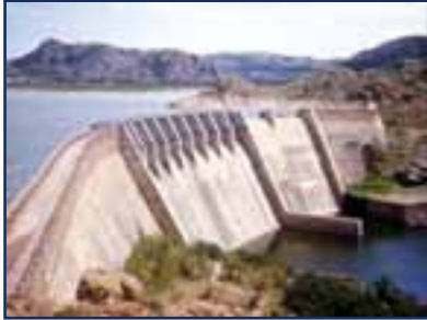
Altus Dam, 1986. The W.C. Austin Project is the first and only reservoir irrigation project in the State of Oklahoma. Photograph courtesy of Bureau of Reclamation, Denver, Colorado.
