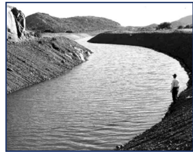
A view of the Main Canal extending southward from Lake Altus, circa 1947. Photo courtesy of the Museum of the Western Prairie, Altus, Oklahoma. Used with permission.
