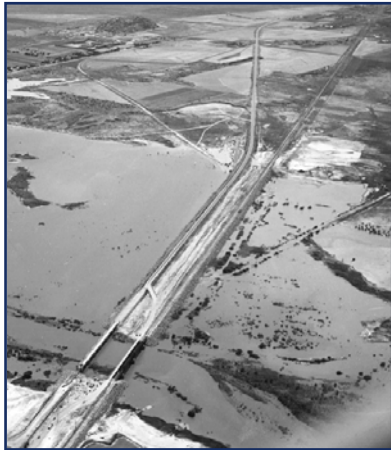
View of ongoing reconstruction of Oklahoma State Highway No. 9 bridge across the upper end of Lake Altus, July 7, 1947 (National Archives and Records Administration 1947b). The earthen approaches of this bridge constrict the lake and have effectively separated the reservoir into two pools, one upstream (right) and one downstream (left) of the crossing.
