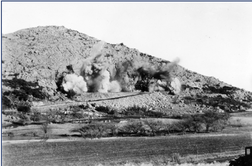
First telephoto shot of large blast of the rock quarry used to supply the granite for the construction of Altus Dam, December 16, 1940.
