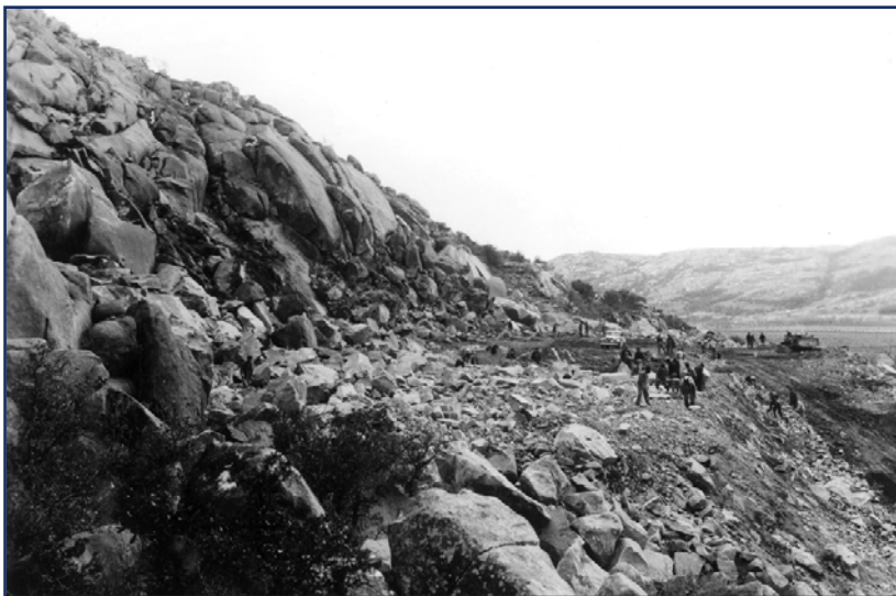
Photograph of rock quarry after the blast, December 17, 1940.
