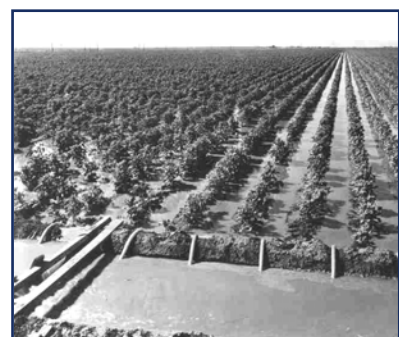
Flood irrigation of a cotton field outside Altus irrigated by water from Lake Altus, circa 1947. Aluminum siphons (foreground) were used to draw water from the canal into the fields. Photo courtesy of the Museum of the Western Prairie, Altus, Oklahoma. Used with permission.
