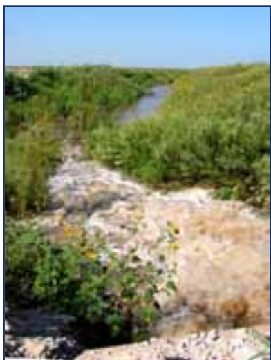
Excess irrigation water being diverted into the wasteway at the end of the Altus Canal, July 16, 2004. The flow rate at the time of the photograph was estimated to be about 50 cubic feet per second. Photograph courtesy of Bureau of Reclamation, Austin, Texas.
