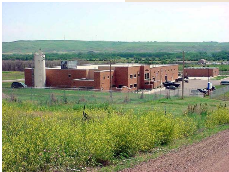
The Mni Wiconi Rural Water System water treatment plant in South Dakota.
