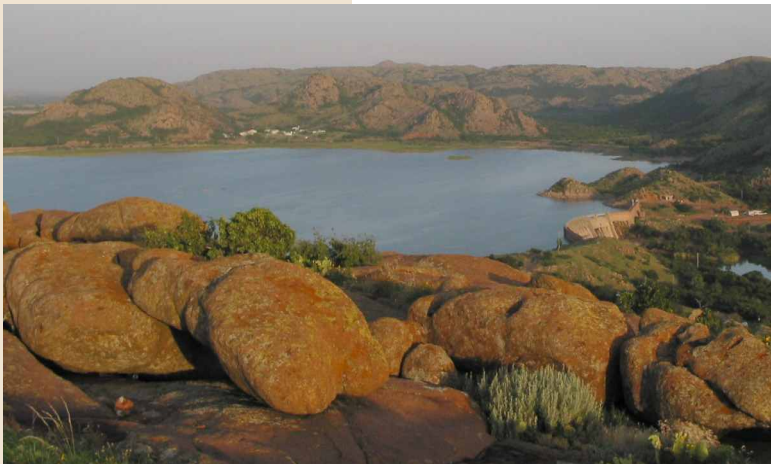
Altus Dam is the storage feature of the W.C. Austin Project.
