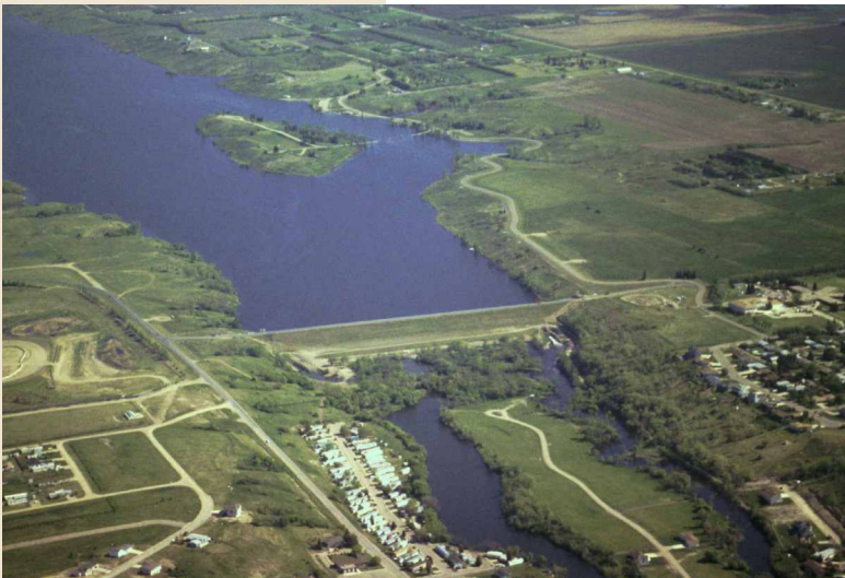
Jamestown Dam and Reservoir.
