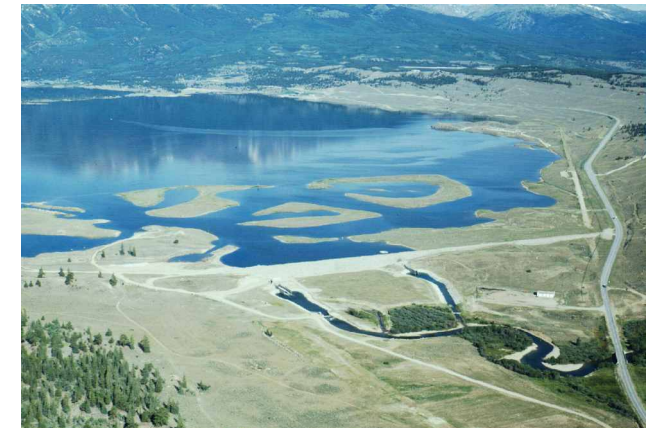
Twin Lakes Dam
