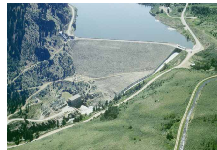
Green Mtn Dam & Powerplant
