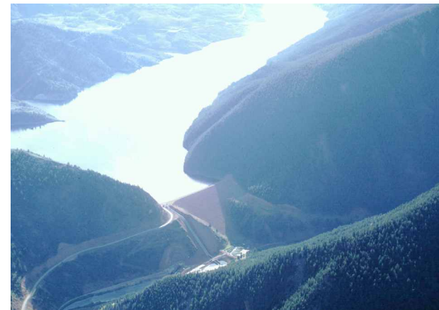
Ruedi Dam (west slope feature)
