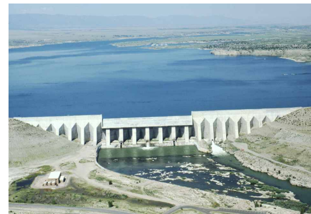
Pueblo Dam & Reservoir
