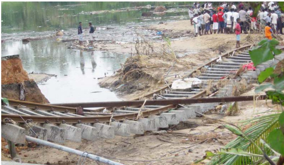
Figure 12. Heavily-damaged southern railway near Akurala.
