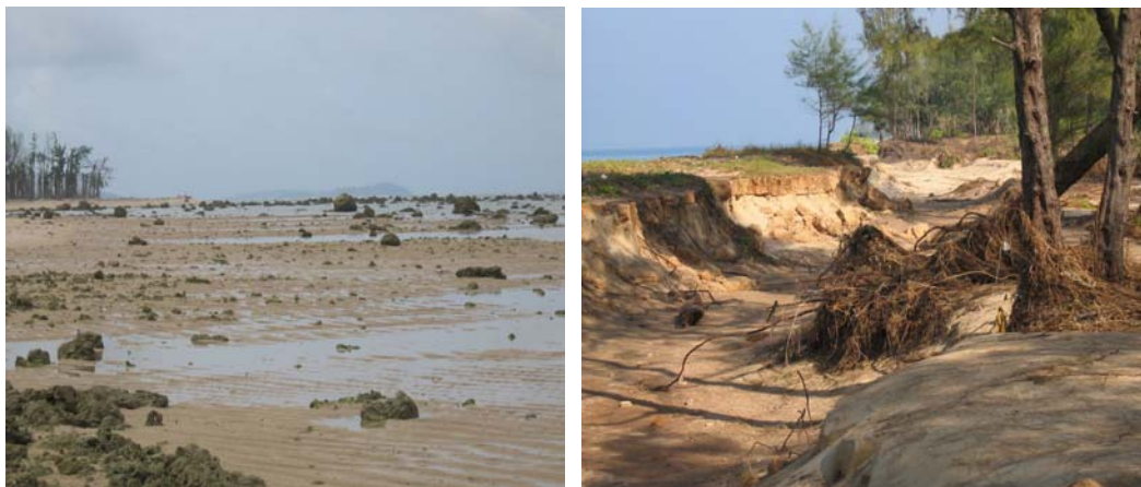
Figure 4 Views of the coastal shores in Takua Pa District after the 2004 tsunami.
