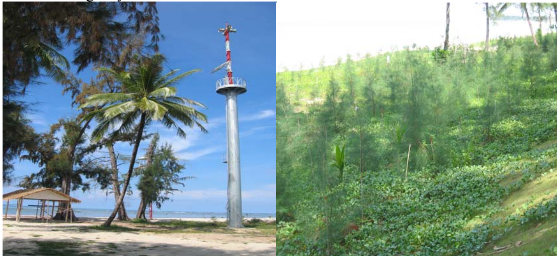
Figure 6 A tsunami warning tower (left) and re-planted beach forests (right) along the coastal shores.
