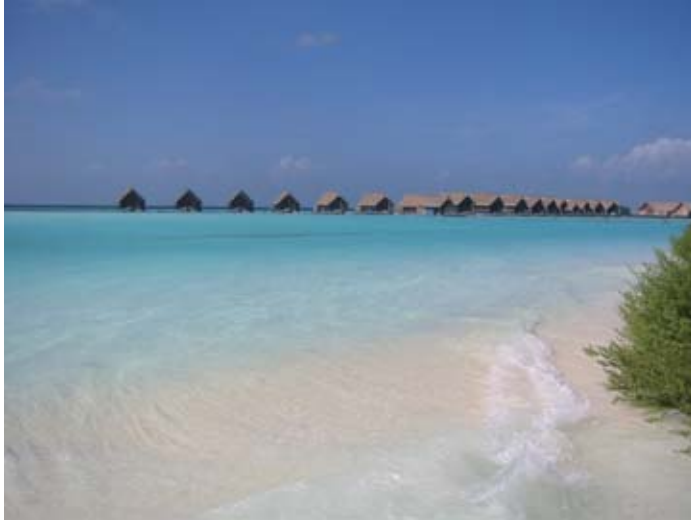
Figure 19. These are the bungalows built on concrete poles within the Cocoa Island resort lagoon. The walkways and the bungalows survived with very little damage. Fortunately the tsunami only reached the base boards of the bungalows, leaving the structures intact.
