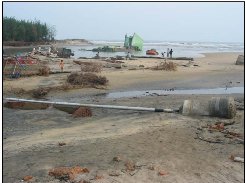
Figure 3: Depicts the damaged children’s park, uprooted electric pole, damaged SINGNADH and the collapsed auditorium on Nagapattinam Beach.
