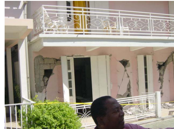
Figure 3. Houses damaged by the earthquake at Petites-Anses, Terre-de-Bas Island (Les Saintes, Guadeloupe; Photographs by N. Zahibo and A. Yalçiner).
