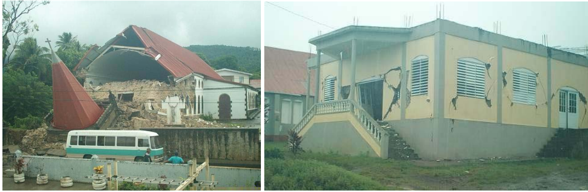
Figure 4. Roman Catholic and Methodist Churches at Portsmouth, Dominica damaged during the earthquake (Wayne Abraham, http://dominicapsn.freeyellow.com/gallery.html ).
