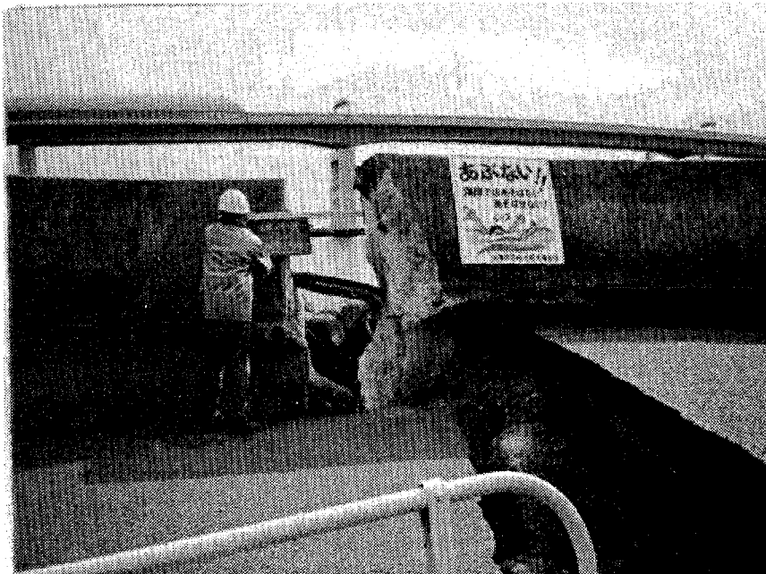
Photo 1 Damage to Coastal Dike in Ashiya Port
