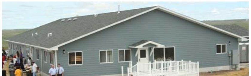
Pictured above is the newly constructed shelter.
