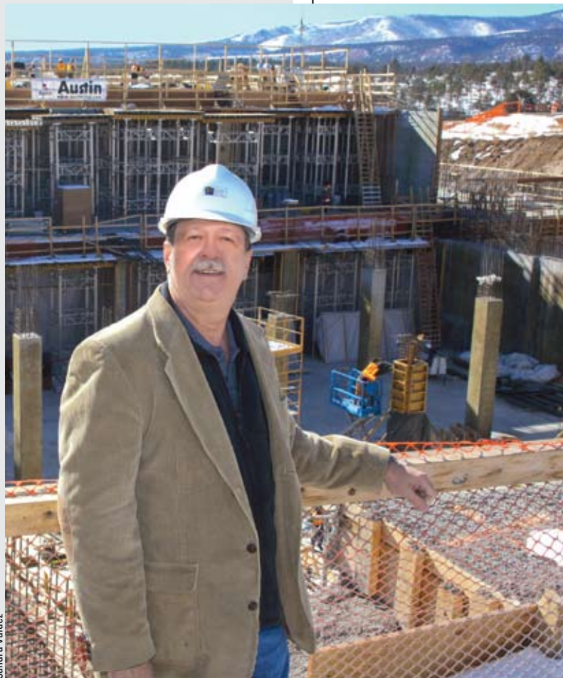
Glenn Mara stops by the Chemistry and Metallurgy Research Replacement Project construction site.
