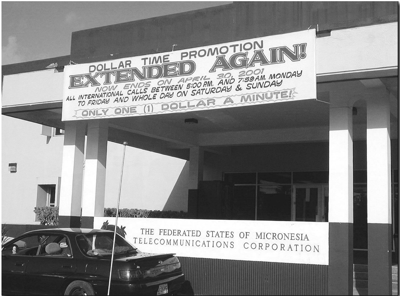
Figure 12: FSM Telecommunications Corporation Building Exterior, Pohnpei, FSM
