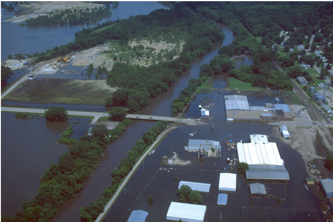
Flooding in Des Moines, IA (photo courtesy of A. Booher/FEMA)
