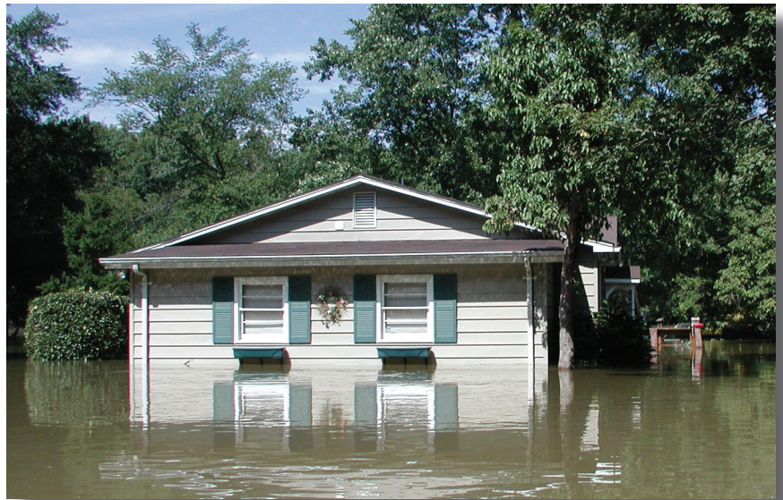
Flooding in Mecklenburg County, NC (photo courtesy of Mecklenburg County)
