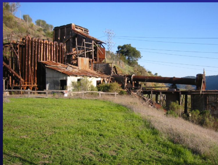
Rotary Furnace installed near Mine Hill in 1940 to increase output of mercury flasks to market
