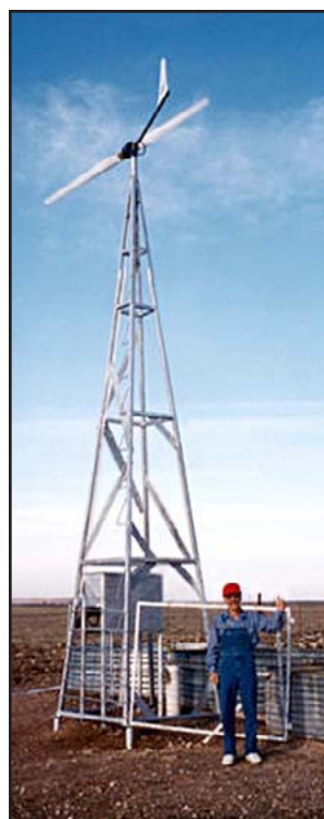
This 1-kW wind turbine from World Power Technology, Inc. is used for pumping water for 120 head of cattle at a ranch in Texas. Source: World Power Technology.
