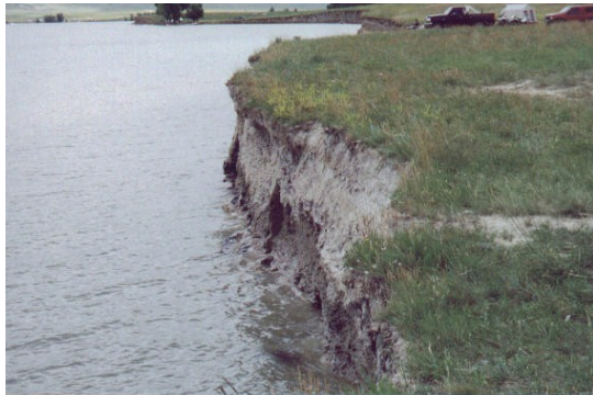
Bank erosion caused by wave action, Belle Fourche Reservoir, 1999
