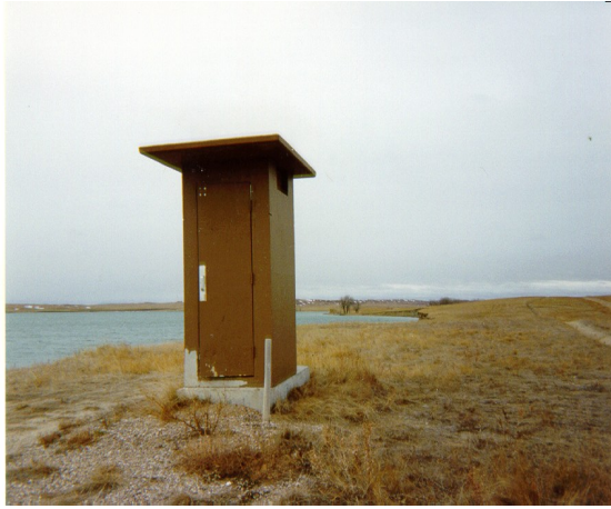
Outhouse located at the end of Gaden's Point
