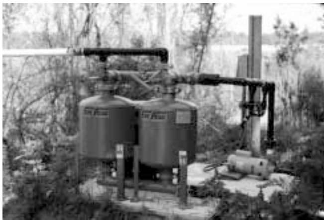
Sand filter, pump, and fertigation unit
