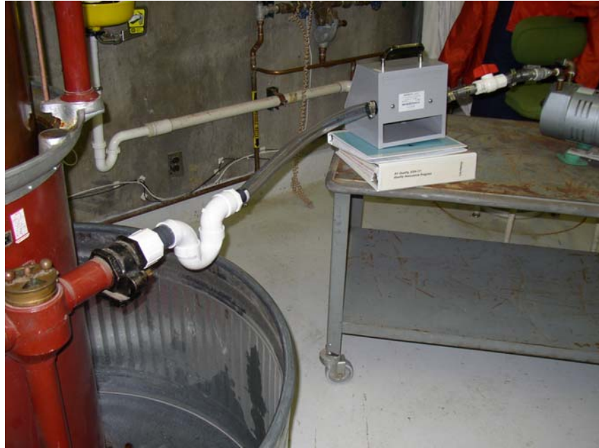
Connection of hoses from bell prover to pump.
